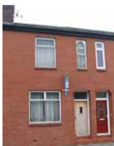
45 Chisholm Street, Openshaw
