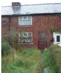
409 Station Road, Winsford
