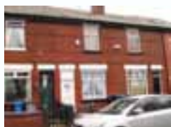
Barlow Road, Levenshulme
