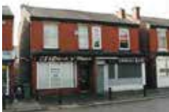
Bury Old Road, Prestwich
