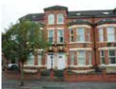
42-44 Lansdowne Road, Crumpsall
