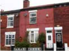
Parsonage Street Heaton Norris
