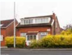
Moston Lane Moston
