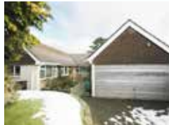
Barlow Wood Road Marple
